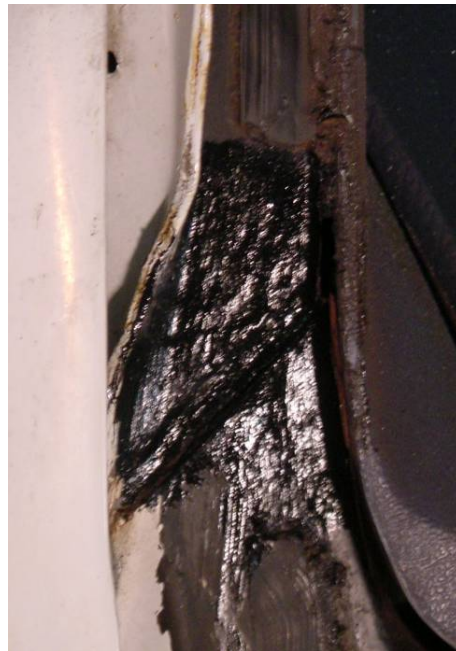
(Same area treated using treatment process)
